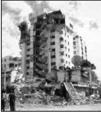
Fig. 3.3a: Destruction caused by an Earthquake at Bhuj
