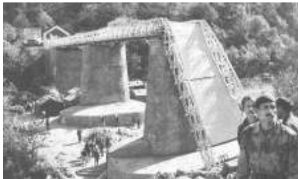
A view of the damaged Aman Setu at the LOC in Uri, due to an earthquake
